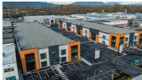
64,572 SF Over Two Buildings WESMONT YALE CENTRE 2138 Carpenter Street, Abbotsford, BC
