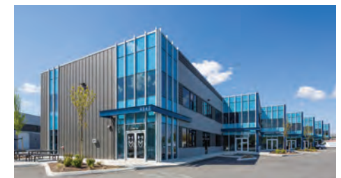
82,472 SF Over Two Buildings PORT KELLS CENTRE 9347 & 9339 200A Street, Langley, BC
