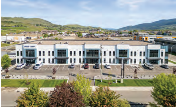
Building A - Exterior and Drone Images
